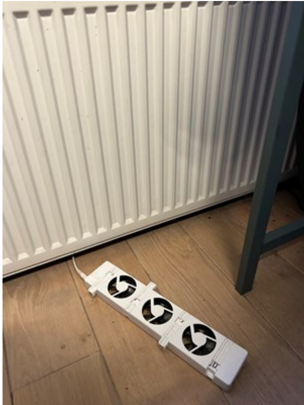
Afb. 9.68 Add-on ventilator
